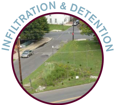
Ferry Avenue Rain Garden: This demonstration project was designed on a vacant lot owned by CCMUA to intercept runoff from surrounding roadways. The completed 900 square foot rain garden can capture, treat, and infiltrate over 75,000 gallons of stormwater each year. | Photo courtesy of CCMUA
